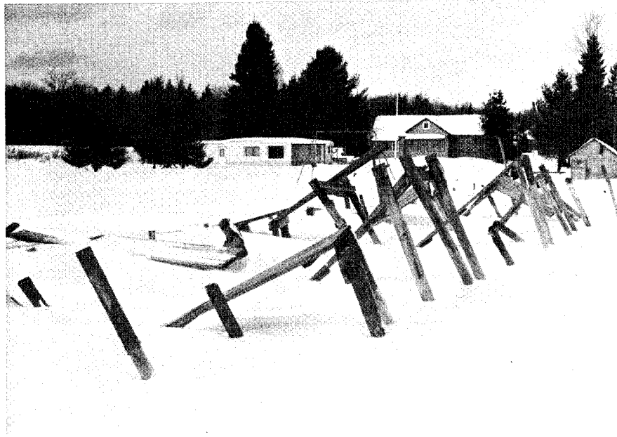
Figure 10. Series of finger piers damaged by ice jacking.
