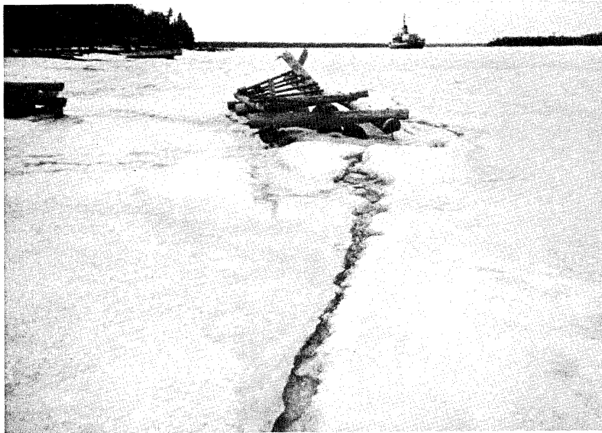
Figure 13. Active crack passing through a damaged dock.
