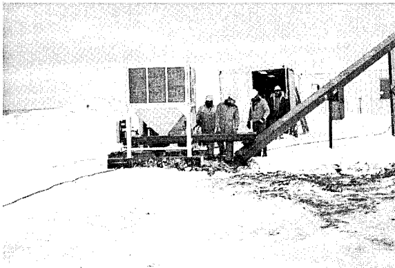
Figure 4. SOUND personnel assembling enclosed lime feed system.
