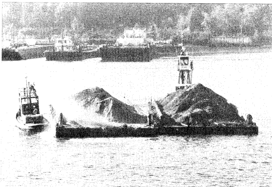
Figure 3. Placement in Area 2 using a high-pressure water jet
