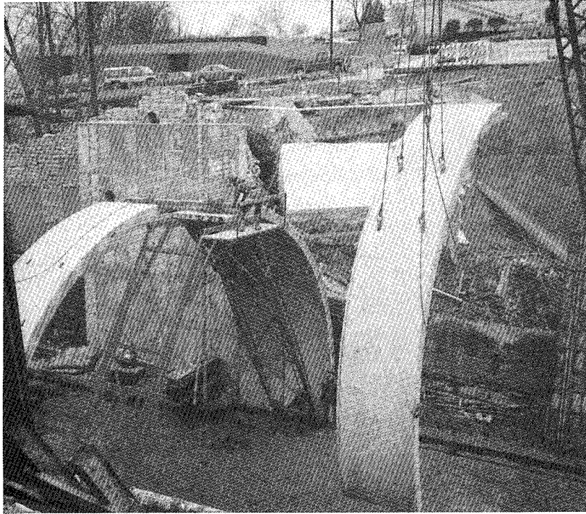
Figure 179. Precast arch sections being installed at Wears Creek (from Hurd 1990)
