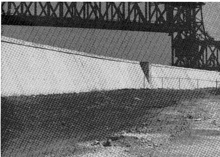
Figure 101. Completed rehabilitation, Joliet Channel Wall
