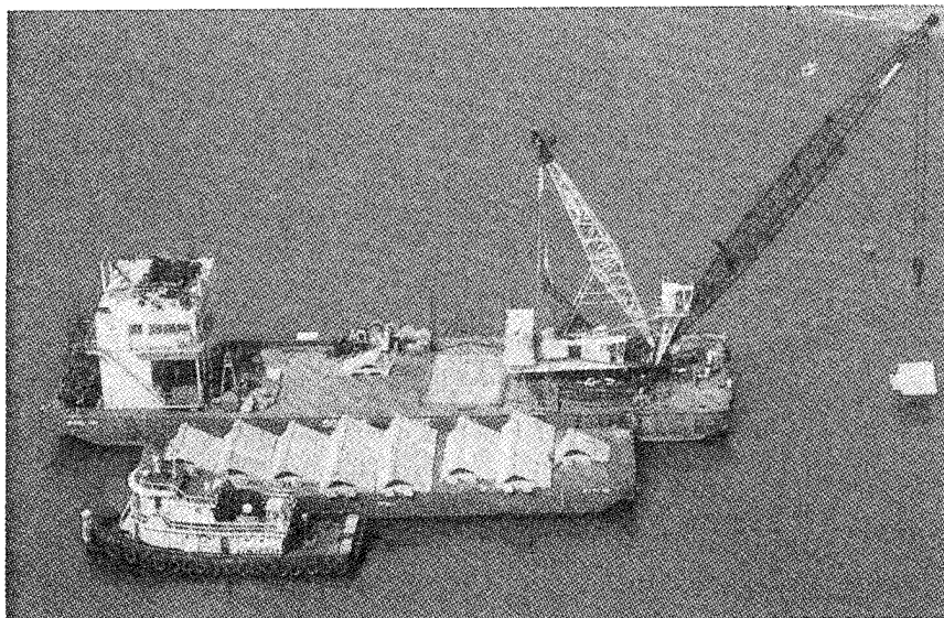
Figure 125. Beachsaver reefs being placed at Avalon Beach (from ASCE 1993)
