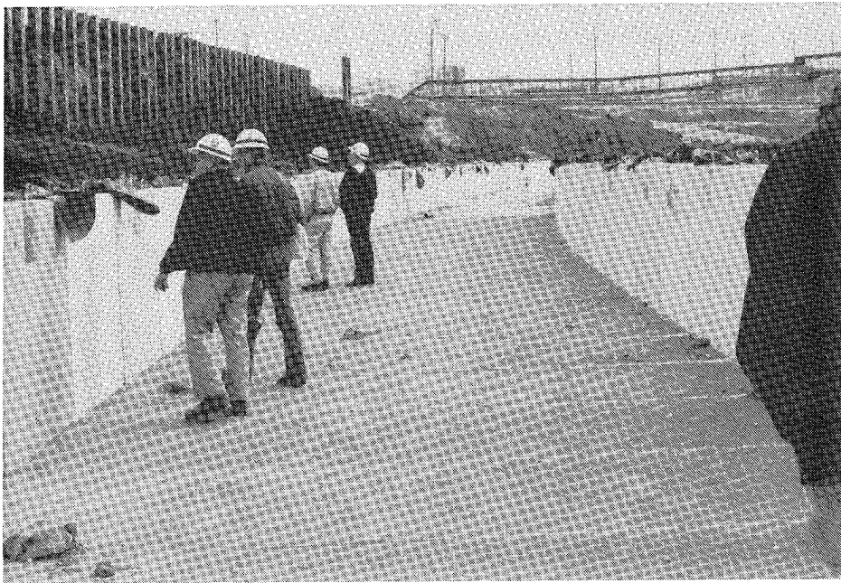
Figure 87. Channel sections in place, Blue River Channel
