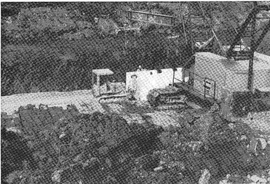
Figure 86. Channel section delivery and installation, Blue River Channel
