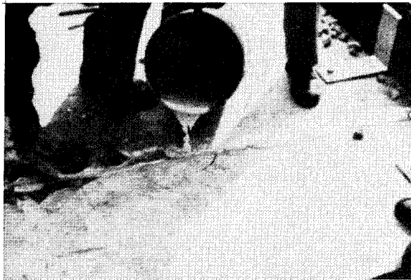
Figure 193. Sand-epoxy grout was used to fill traverse joints between the slabs on the Santa Fe Railroad redecking (from Hyma 1979)
