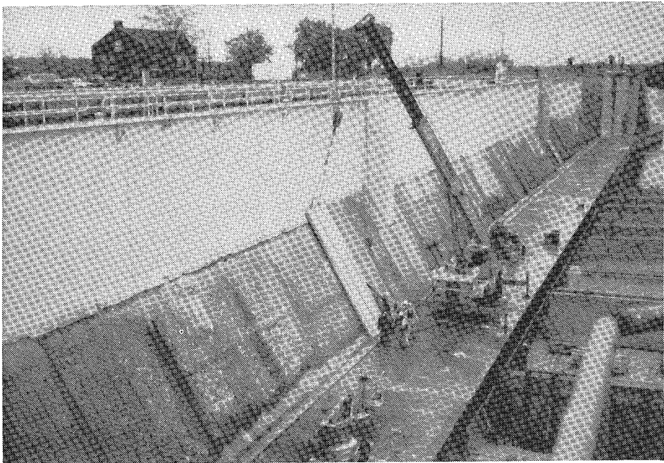
Figure 26. Completed river wall repair, Lockport Lock
