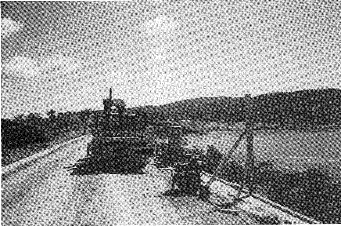
Figure 53. Upstream and downstream footings for precast panels, Googong Dam
