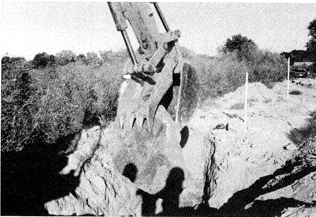
PHOTO NO. 6. BLOCK SAMPLE FROM STA. 0+50
