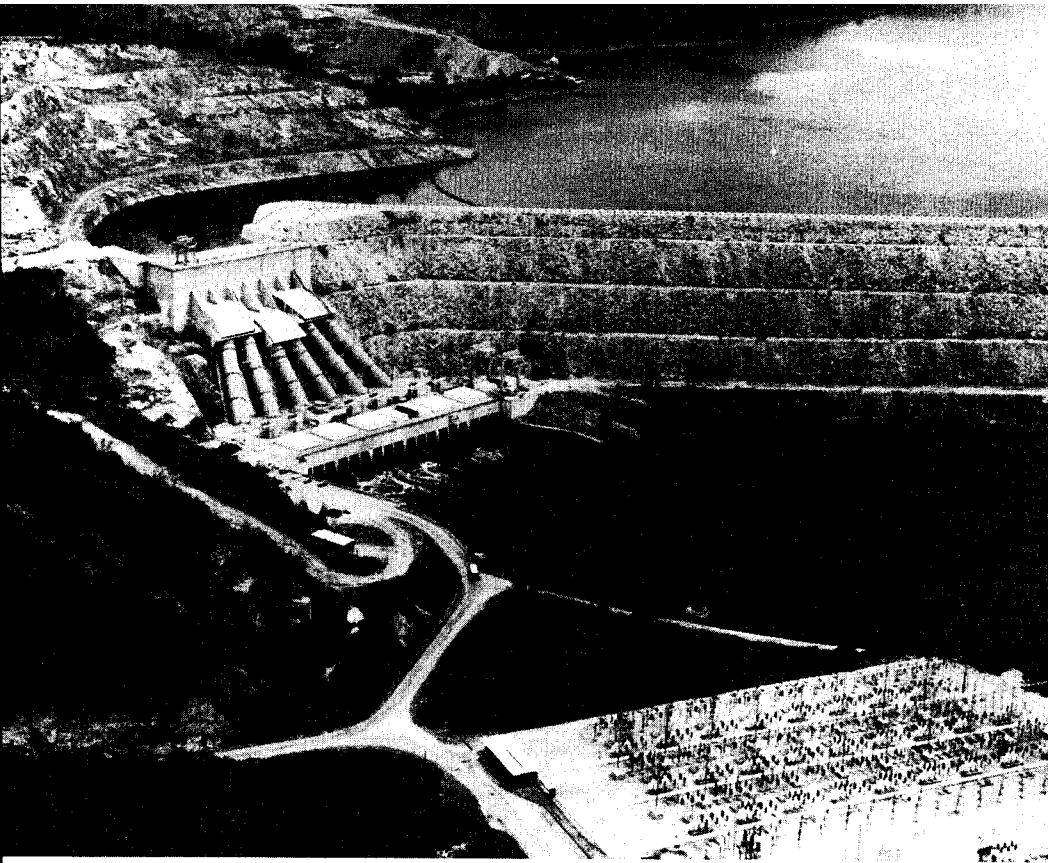
Hydroelectric sluices in the Akosombo Dam Courtesy Embassy of Ghana, Washington
