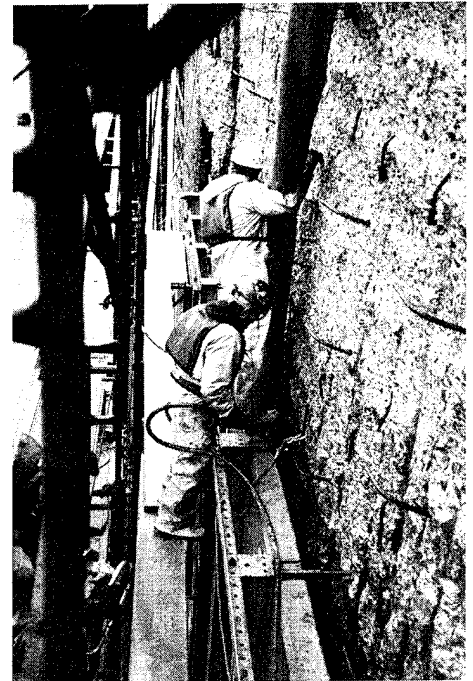
Figure 8. Flexible elephant trunk concrete chute
