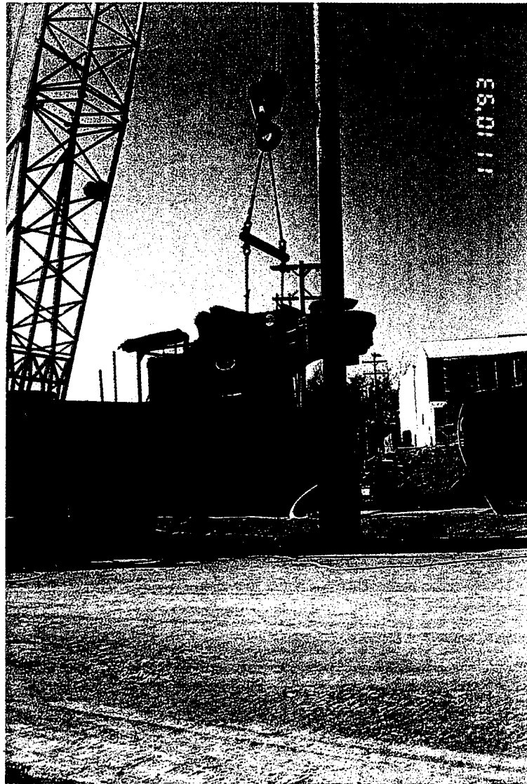
Crane LINK BELT LS338 equipped with rotary table for driving bucket (November 1993)
