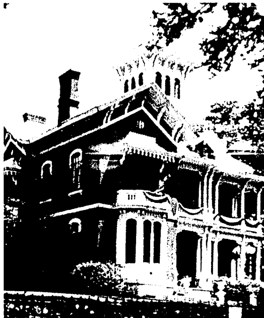
2. Nineteenth century buildings continued to use architectural features such as porches, cupolas, and awnings to make the buildings more comfortable in summer, but heating was greatly improved by hot water or steam radiators. Photo: NPS Files
