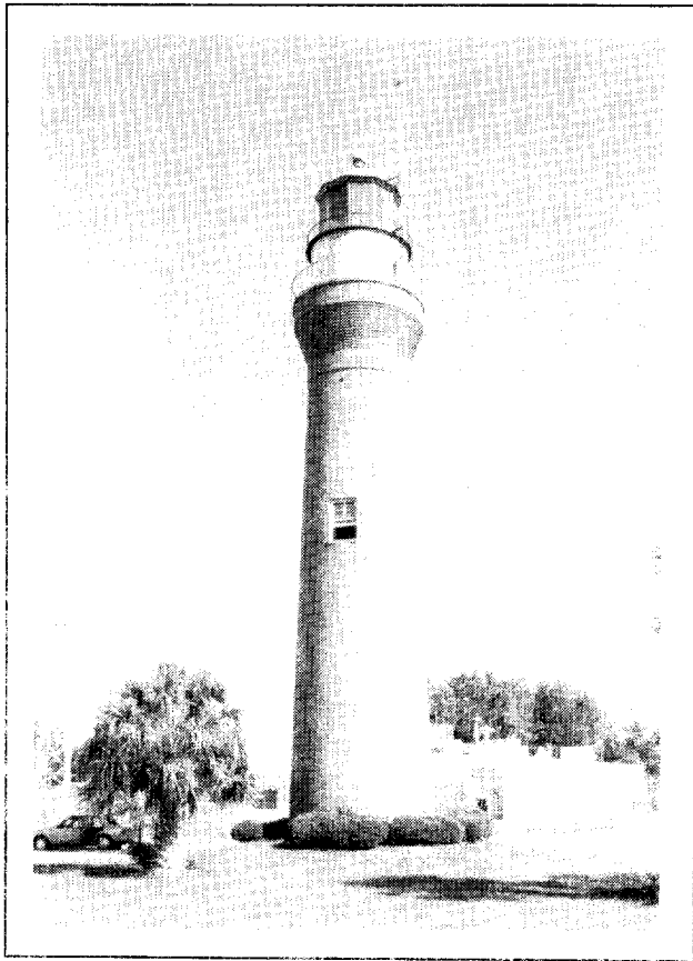
Figure 1. St. Johns River Lighthouse site.
