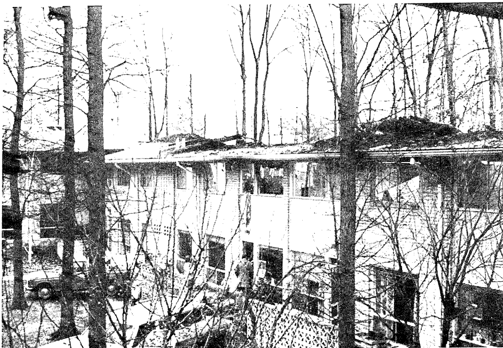
Figure 8. The combustible attic forms a vast horizontal flue.
