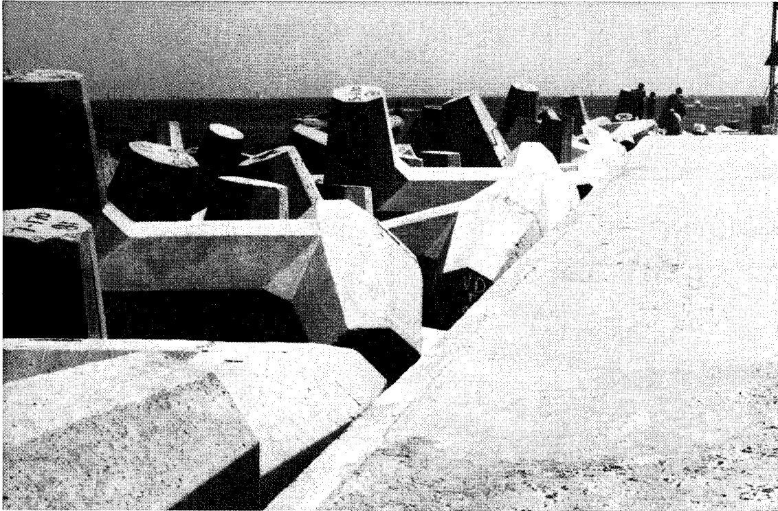
Figure 5. Closer view of 16-ton dolos armor units on the heads of Manasquan Inlet jetties
