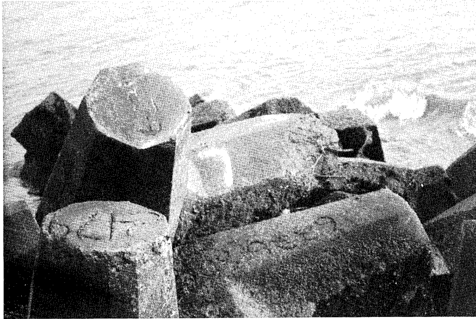
Figure 19. Dolos on south jetty with shank/fluke break
