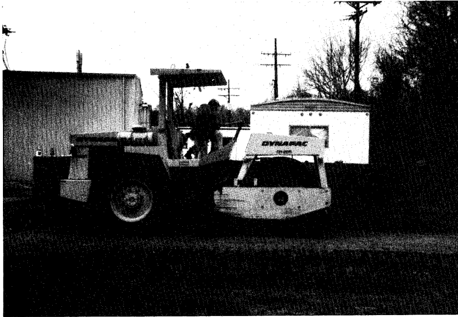
Figure 19. RCC test section constructed at WES
