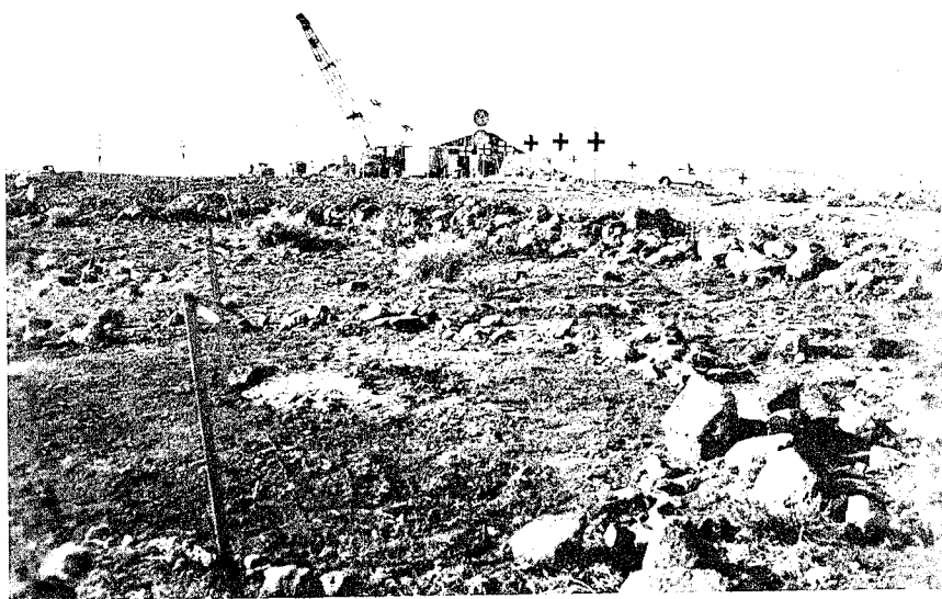
Figure 1.3 Cleared Area Around Gage Installation
