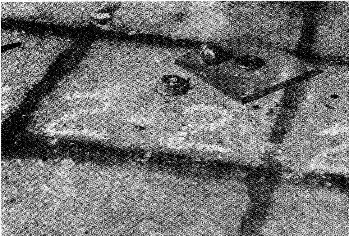
Figure 28. Steel fails before epoxy on encapsulated resin with epoxy filler anchor
