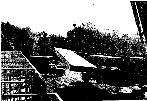
Figure 7.—A factory-built stressed-skin floor panel being moved onto supporting structure.
