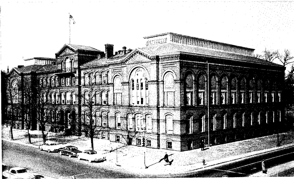
FIGURE 137.—This building, erected for the Army Medical Museum and the Army Medical Library in 1887 was in part occupied by the Museum and its successor, the Institute, until 1955. The Museum and certain offices of the Institute returned to this home in the centennial year 1962.
