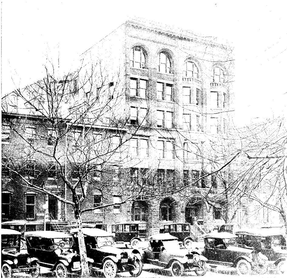
FIGURE 49.—After 15 years of operation in the Museum building, the Army Medical School moved in 1910 to rented quarters on Louisiana Avenue.
