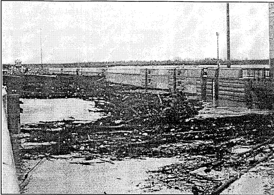
Typical log jam, Lock and Dam Operation
