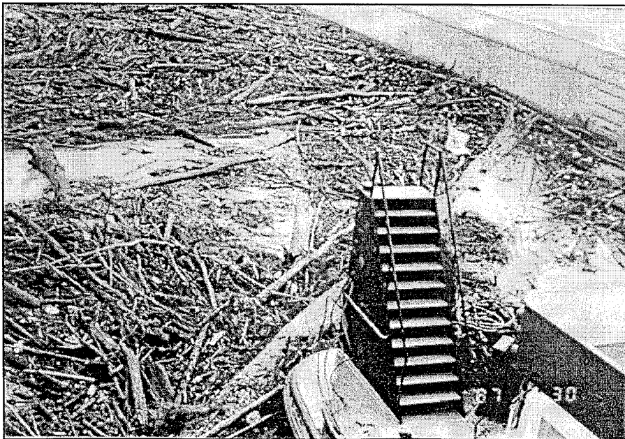
Typical log jam, Lock and Dam Operation
