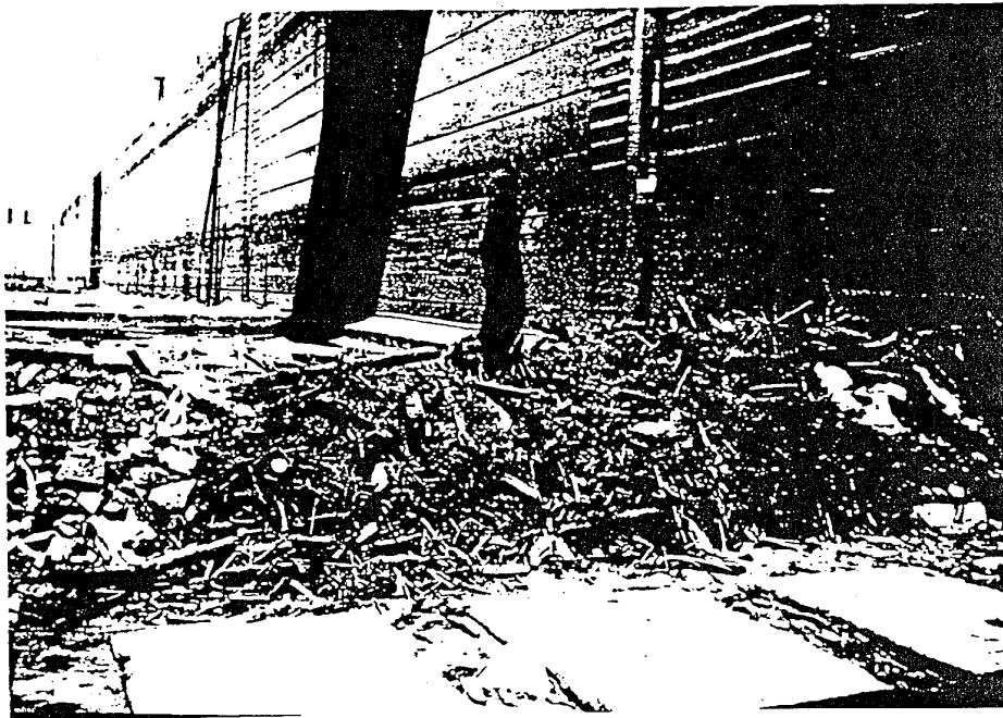
FIGURE D - DEBRIS ACCUMULATION - MARKLAND 600-FT LOCK CHAMBER (view from down in the lock chamber)
