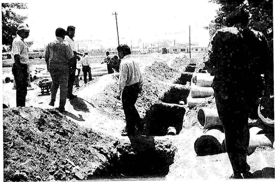
Figure 2.2: CARE Sewer Infrastructure Improvement Food-for-Work Project in Honduras
