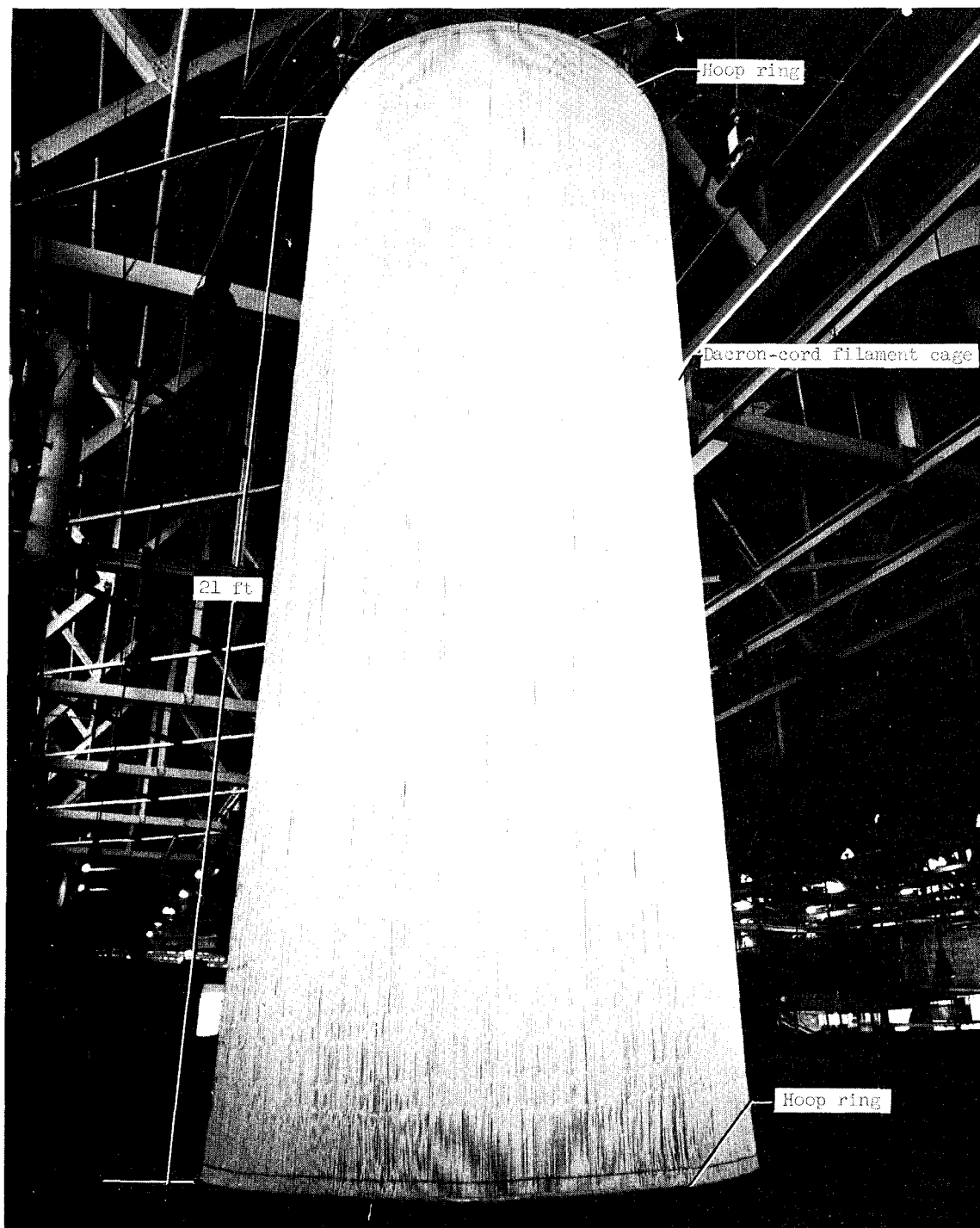
(a) Final filament-cage construction.
