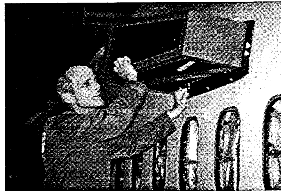
FIGURE 19. UPPER WINDOW BELT INSPECTION
