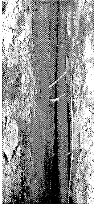
Conduit pipes laid in the ground to meet at an intersection in the pull box. Below: Contents of the plastic pull box.
