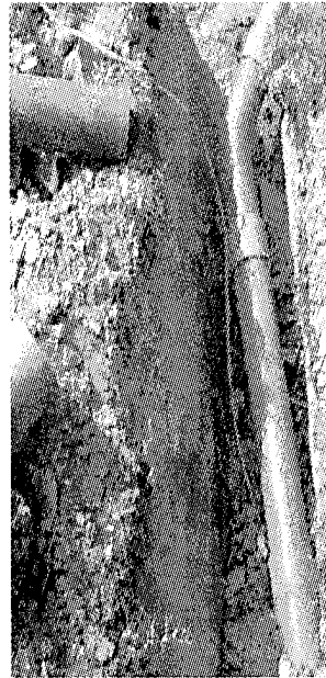
Conduit pipes laid in the ground to meet at an intersection in the pull box. Below: Contents of the plastic pull box.
