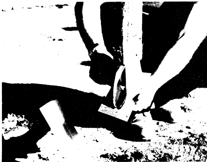
Figure 2. Vertical strip drain installation procedure
