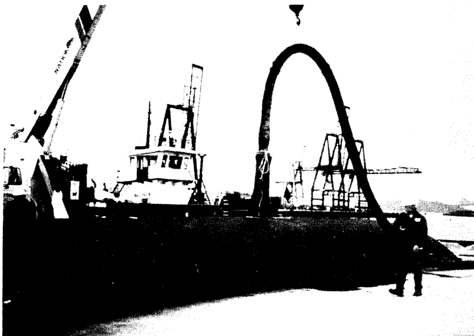
Figure 3. Hydraulic filling of a GFC at the Port of Oakland
