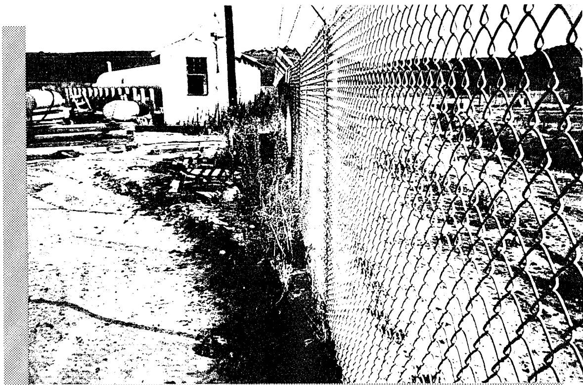
Photograph 1: Old Battery Maintenance Area, located 150m ESE of Bldg. 25012. Neutralized battery acid discharged to culvert seen in right side of picture.
