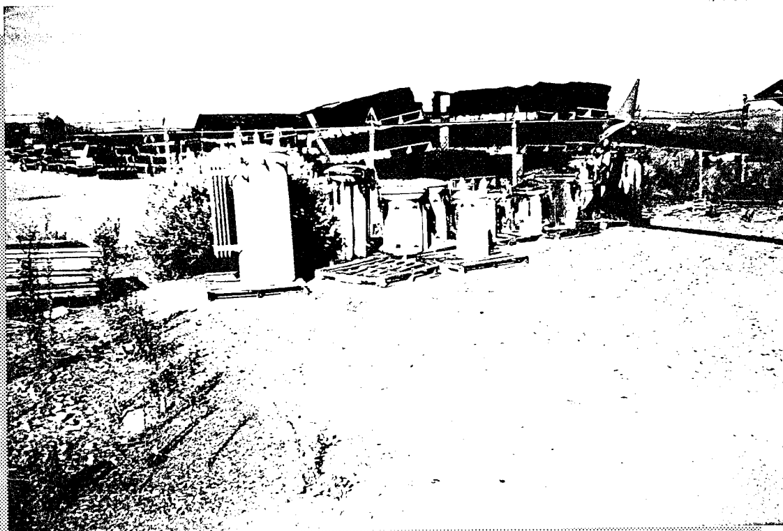
Photograph 16: Old/New PCB Transformers, north of Bldg. 6418.
