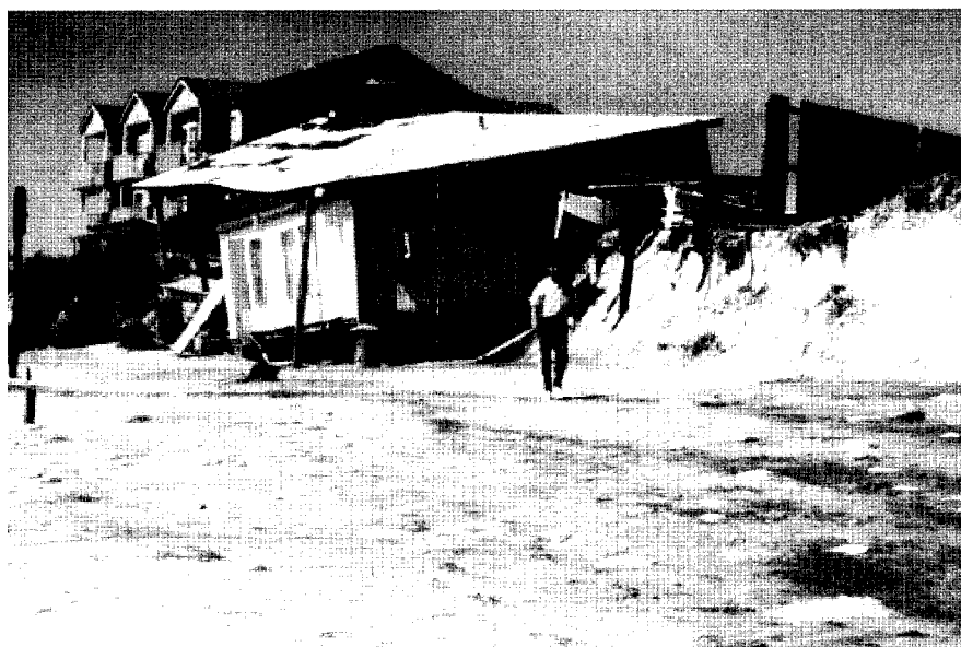
Figure 1. Storm-induced beach erosion produced by Hurricane Opal, October 1995, Walton County, Florida
