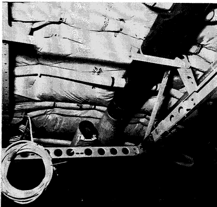
FIGURE A-8. SIDEWALL DROPPERS FROM CENTERLINE DUCT
