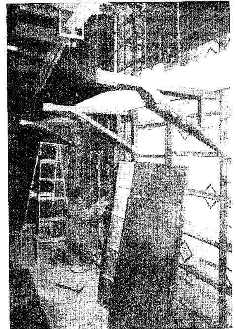
Figure 5. Forming for interior shear walls
