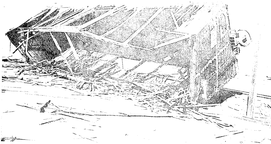
Fig. 4.10 Postshot, Damage to Wooden Boxcar, 3.6f
