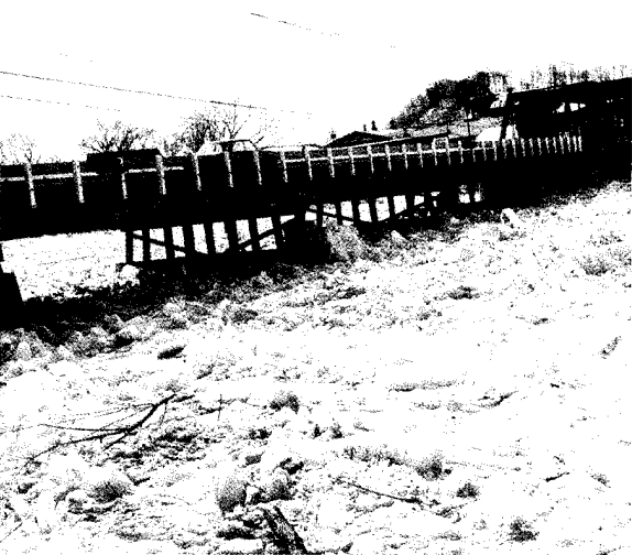
Figure 4. Temporary piers subjected to ice forces in 1969.
