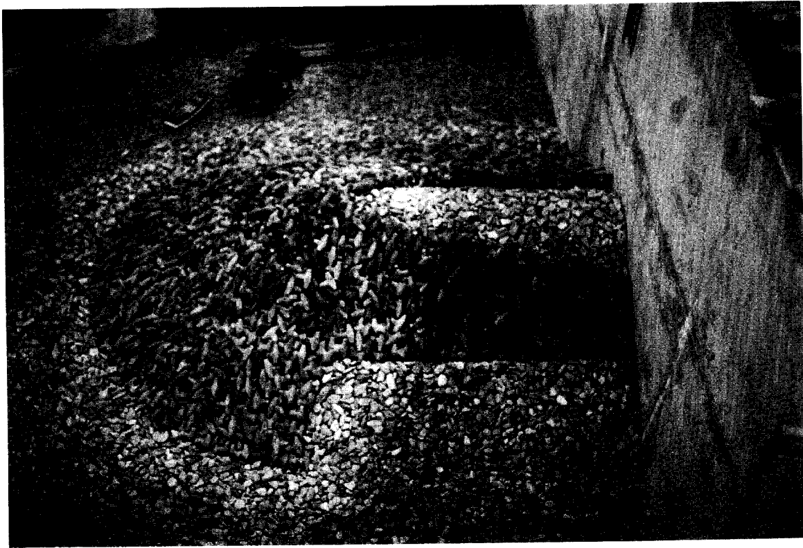
Photo 4. "Inverted V" placement technique for concrete armor units
