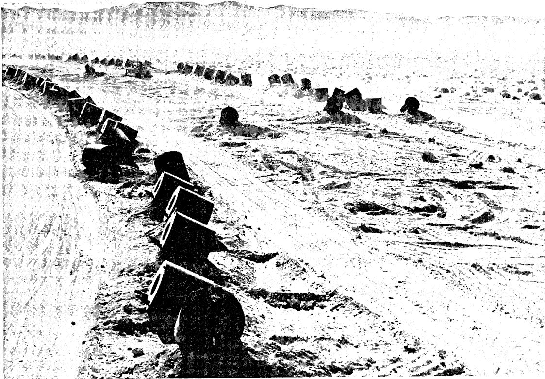
Fig. 3.7—Collimators in place.
