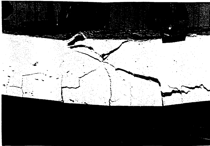
Figure 29. View 1 of Non-Instrumented Rebar Beam Failure Mode.
