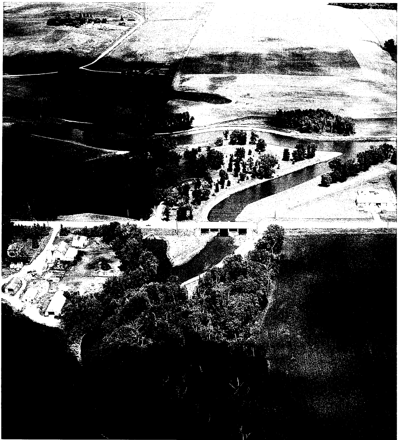
CHIPPEWA DIVERSION DAM LOOKING UPSTREAM
