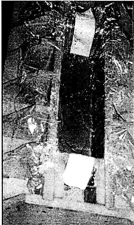
Figure 3-36: Pour Paste in Form
