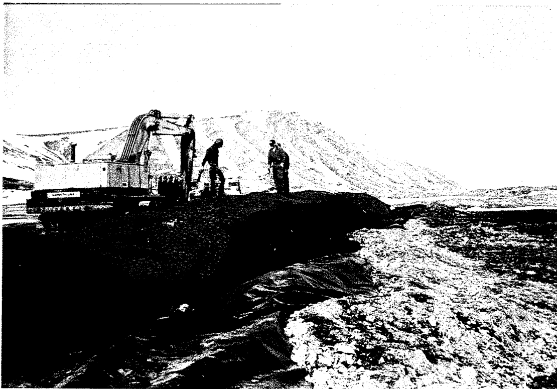
Photograph 21: Prior to installing the containment cell cover, used carpet was laid over the spoils pile to minimize the potential for sharp objects to puncture and tear the cover.
