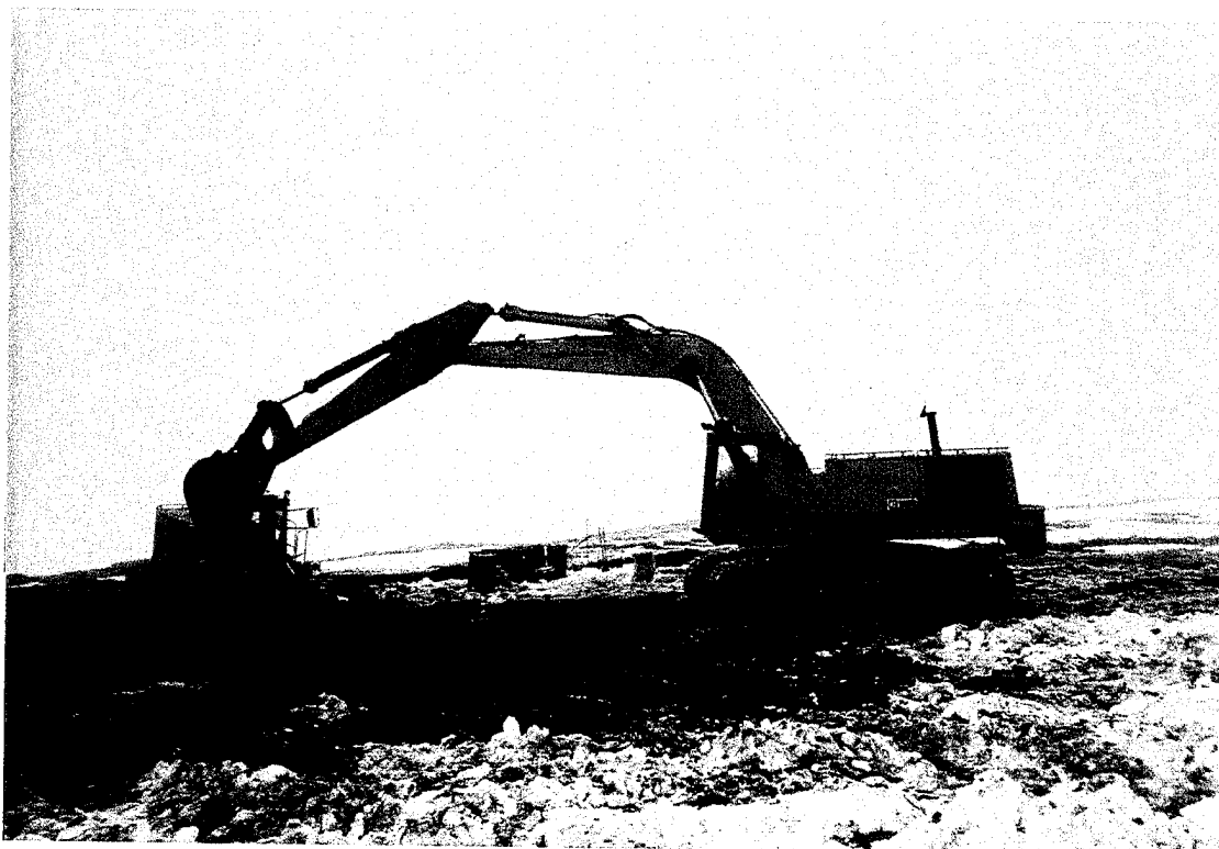
Photograph 8: An excavator was used to remove drums and soils from the pit.
