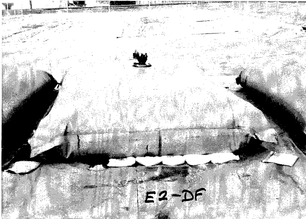
Photograph No. 5. Soiled spill control pillows around E-2 minitank containing diesel fuel
