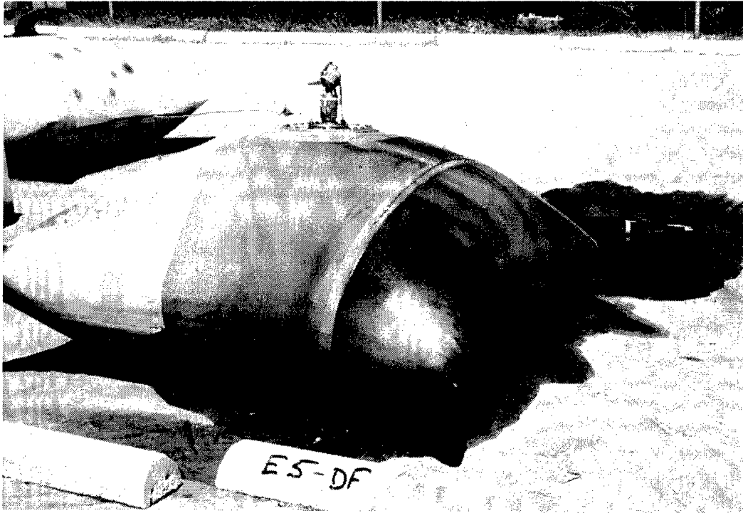
Photograph No. 15. Evidence of E-5 minitank diesel fuel leakage
