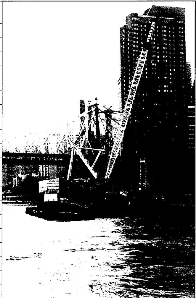
Weeks Marine Inc. Barge Crane
