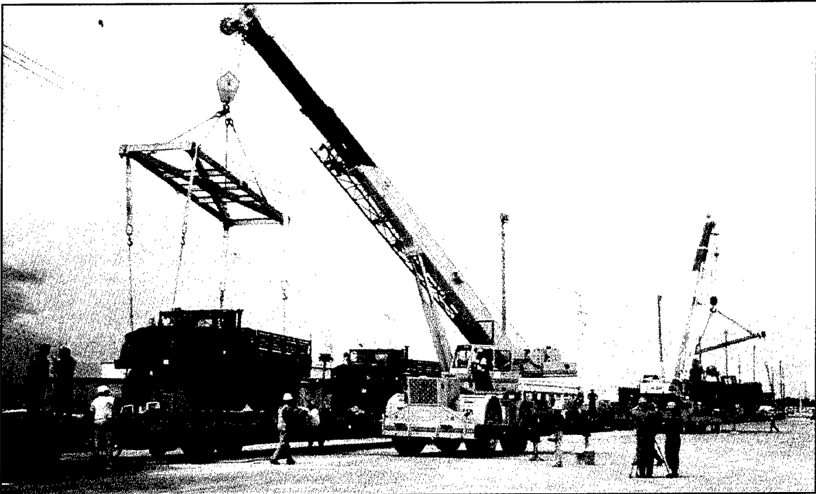
Mobile Cranes at Blount Island
