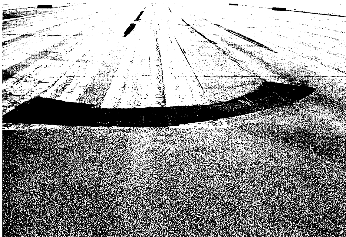
Photo C2. Patch of slippage crack on Runway 13-31
