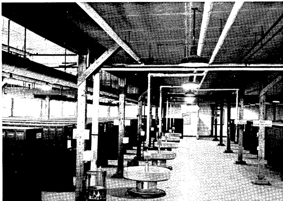
Figure 36. Typical employee locker room at the Twin Cities Ordnance Plant during 1941-1945 (TCAAP Public Information Office).
