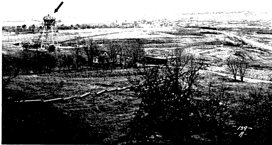
Figure 18. View of Twin Cities Ordnance Plant location during construction. Note Fort Snelling water tower (TCAAP Public Information Office).
