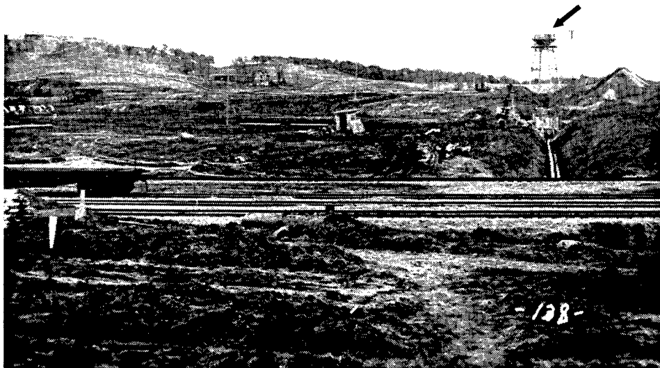
Figure 19. View of Twin Cities Ordnance Plant location during construction. Note Fort Snelling water tower (TCAAP Public Information Office).
