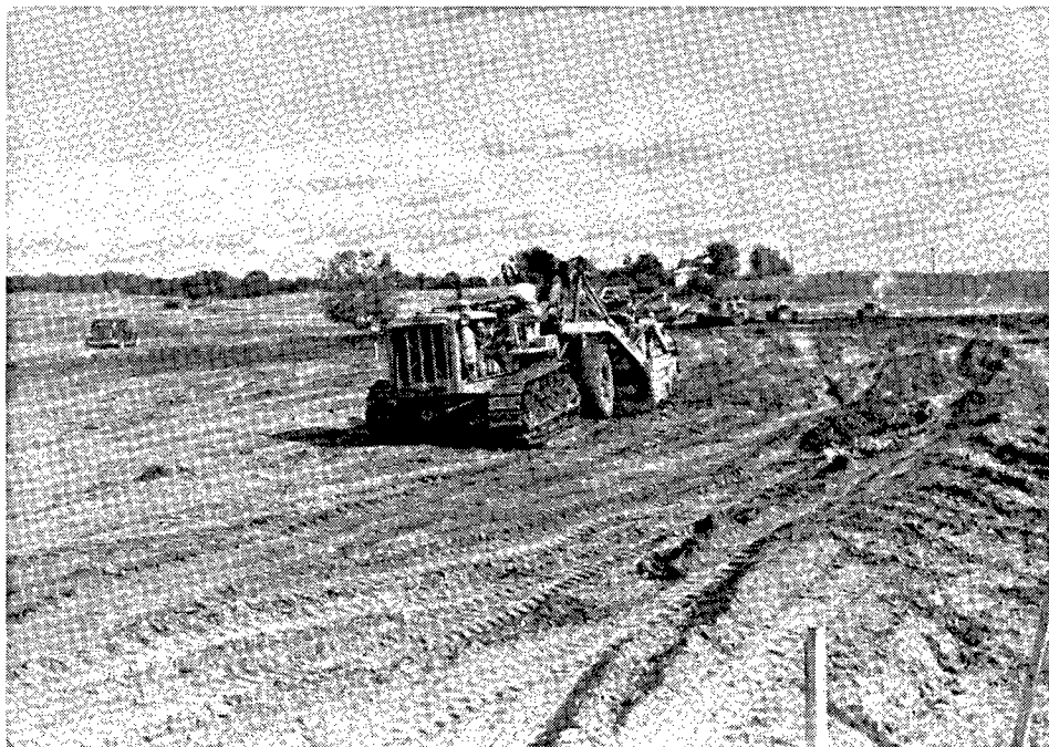
Figure 9. Construction work at the Twin Cities Ordnance Plant. Grading the building site. Minneapolis Star Journal photograph, undated but probably from August 1941 (Minnesota Historical Society).
