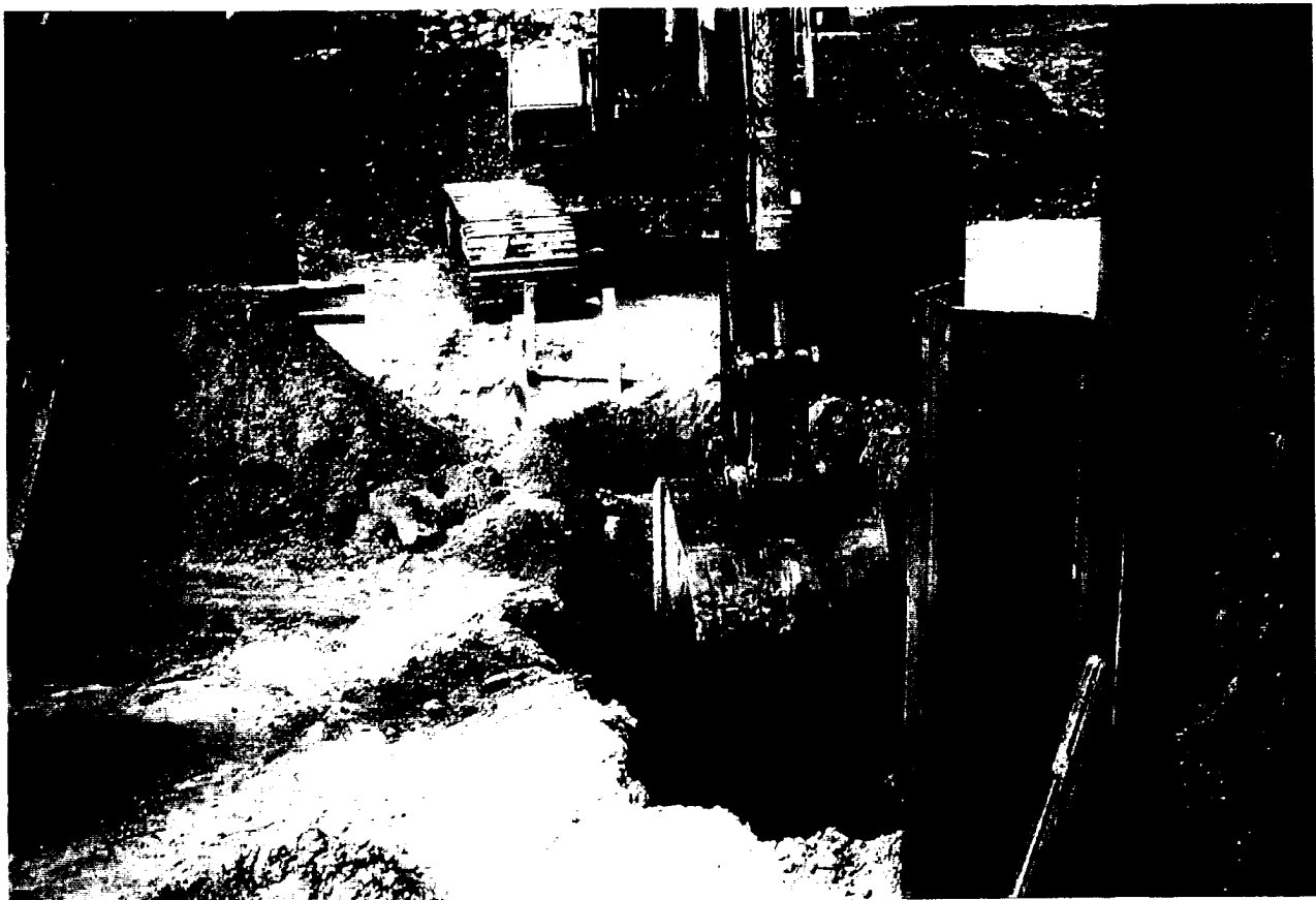
40. Removing Tertiary rock stratum 2 feet below final grade in the upstream guardwall area to allow installation of sheet pile.
