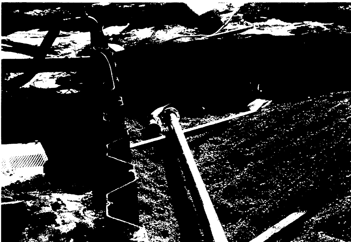
32. Installation of the stainless steel collector system beneath the stilling basin. Note filter materials and sheet piling.
