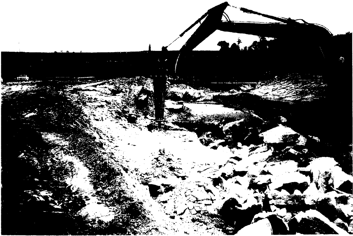
15. Excavating Tertiary rock stratum using hydraulic hammer.
