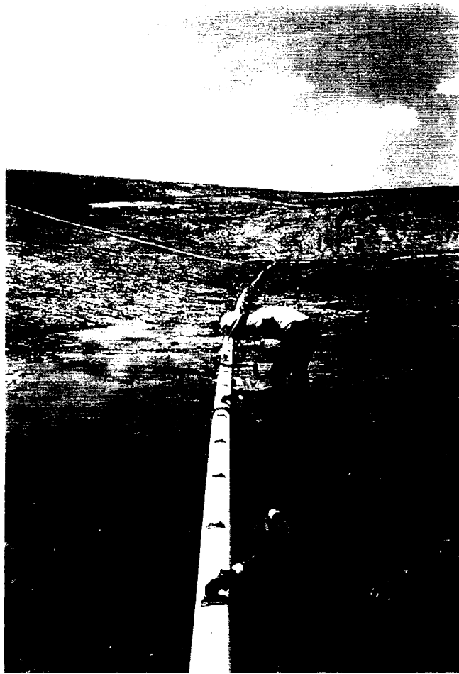
25. Wellpoint system used to lower Tertiary hydrostatic pressures for the gated dam excavation.
