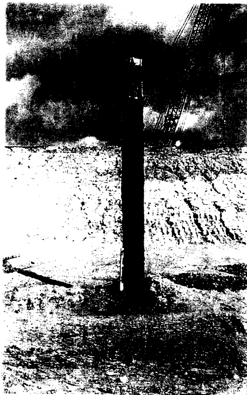
4. Government well used for pump test. Note iron encrusted sand and gravel encapsulating the well screen.
