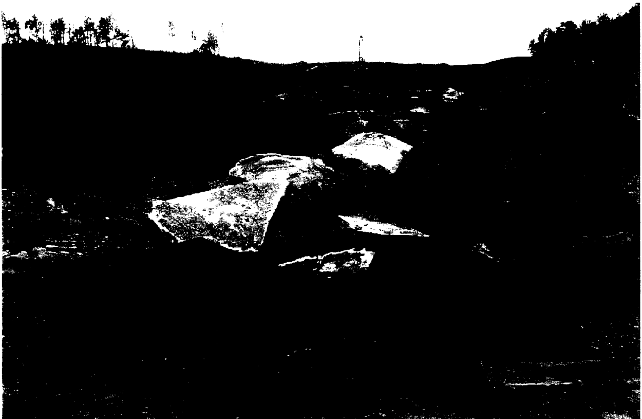
16. Tertiary rock to be transported to the spoil area.
