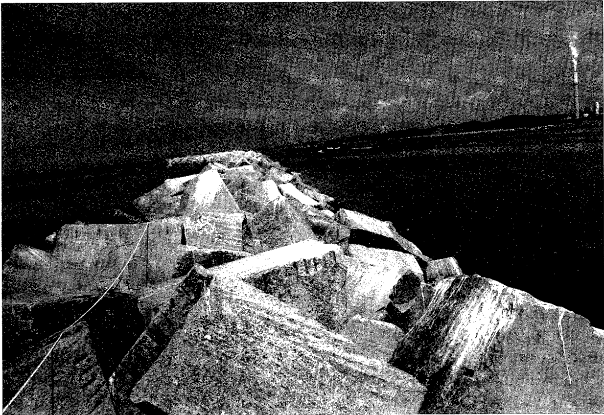
Figure 4. View of armor stone on breakwater trunk
