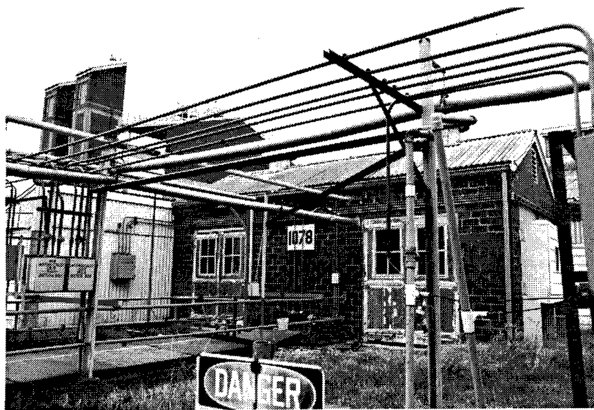
Figure 50. Building 1078: Wash House of the Medium Caliber Loading Buildings.
