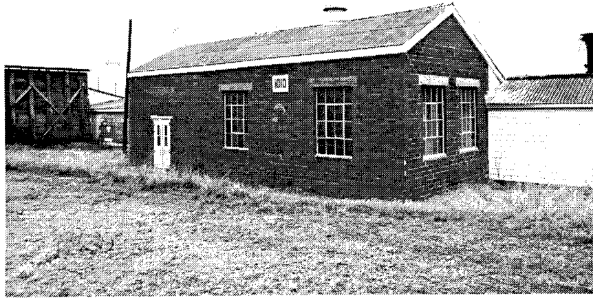
Figure 40. Building 1010: Booster House.
