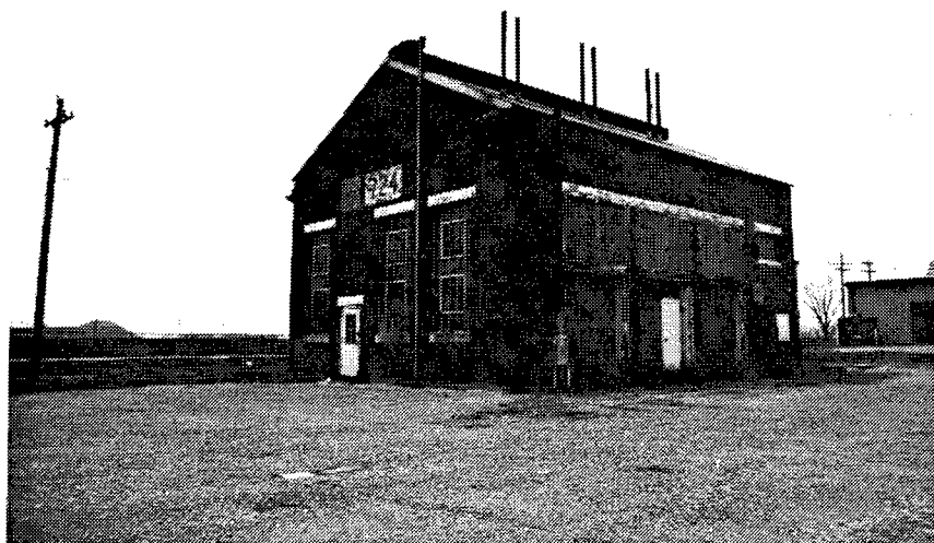
Figure 18. Building 724: Oil Boiler House.
