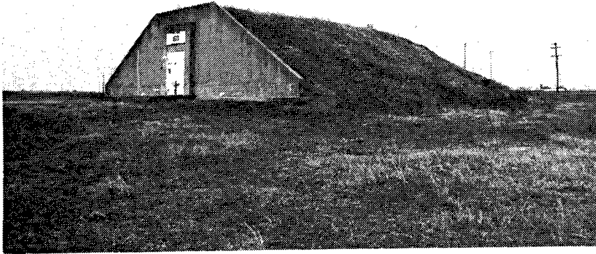
Figure 83. Building 1620: Storage Igloo.
