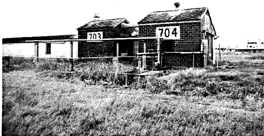
Figure 14. Building 703 (left) and Building 704 (right): A Heater House and an Azide Building, respectively.
