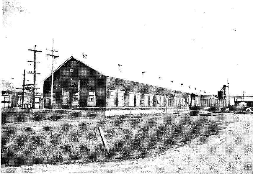
Figure 64. Building 203: Maintenance Shop portion of the General Purpose Administration Building.
