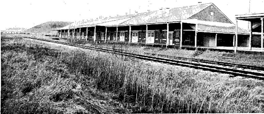
Figure 84. Building 1005: Process Storage Building with earthen berm that was built to compensate for the close proximity between it and other buildings on the line.
