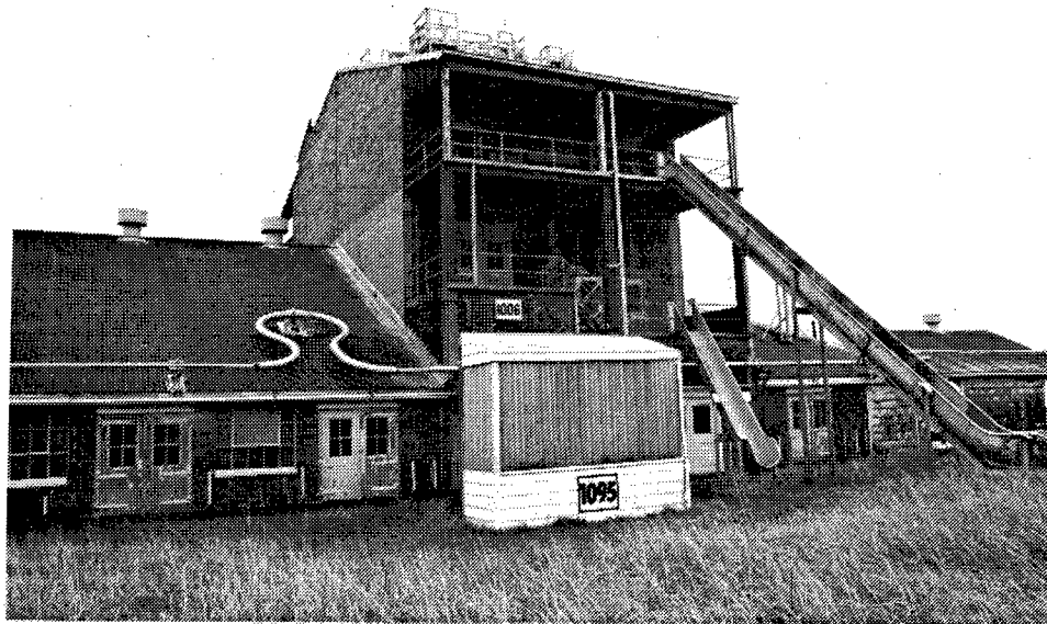
Figure 44. Building 1095: Vacuum House responsible for the collection of loose powder within the line. There are numerous vacuum houses of varying design throughout the 1000 line.
