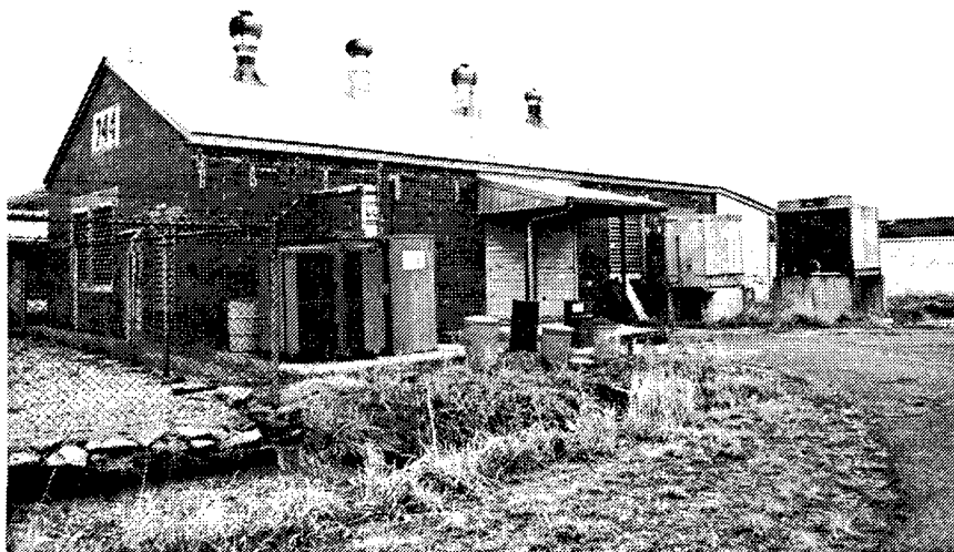
Figure 21. Building 744: Compressor House.
