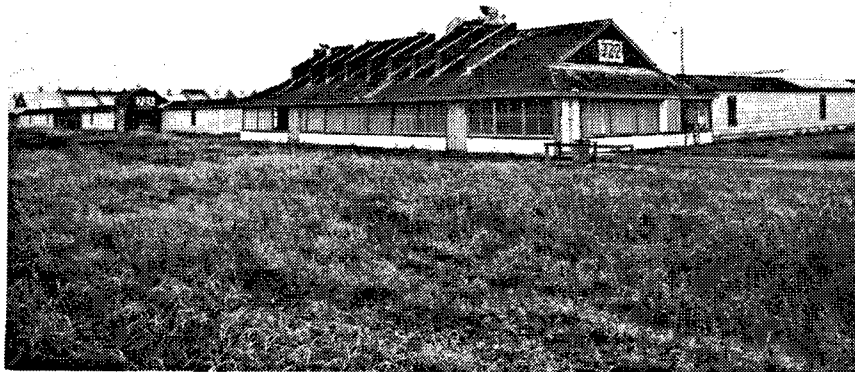
Figure 17. Building 722: Detonator Rumbling Building which has recently served as a Detonator Lacquering (painting) Building.
