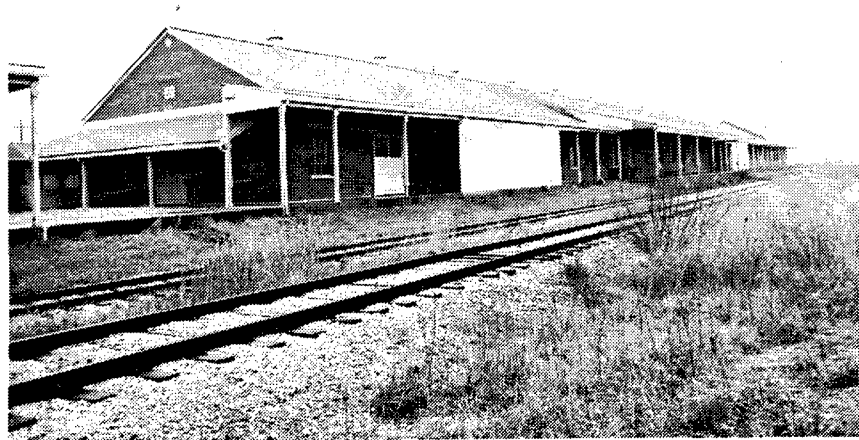
Figure 76. Building 1003: General Purpose Warehouse - Process Storage.
