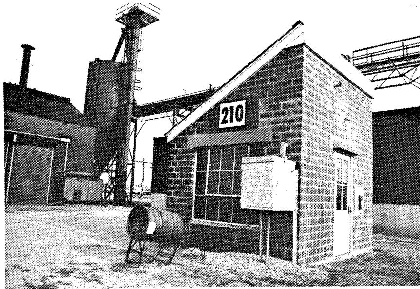
Figure 99. Building 210: Pump Station Building.
