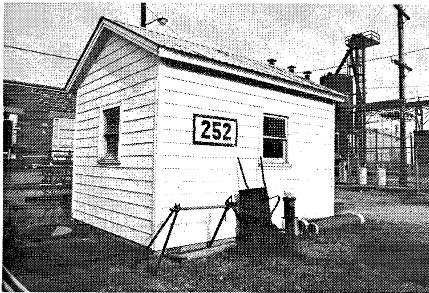
Figure 74. Building 252: Lumber and Pipe Shed.
