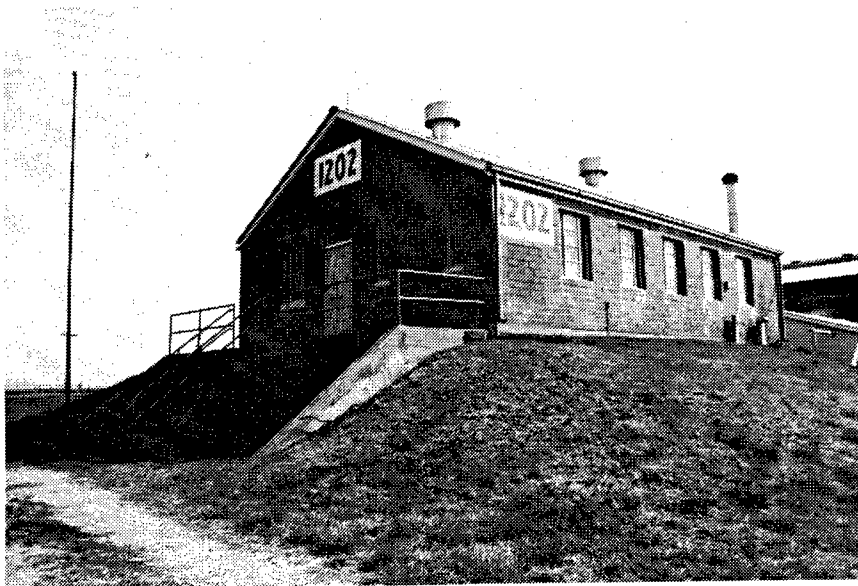
Figure 93. Building 1202: Change House in which the design differs from those on other lines.
