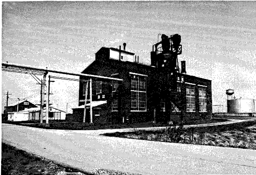
Figure 54. Building 1205: Coal Boiler House located on the 1200 Line that served as the Ammonium Nitrate Plant Modifier.
