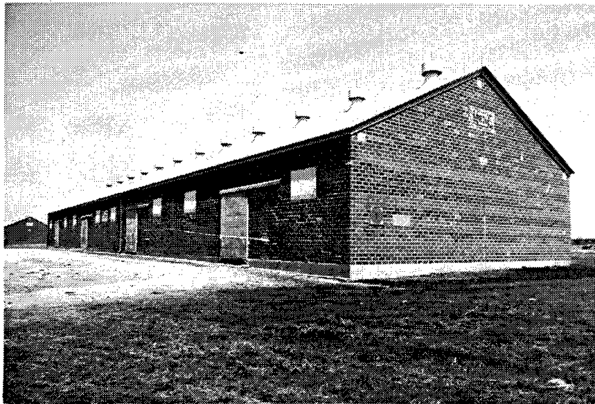
Figure 82. Building 1826: Finished Ammunition Magazine.
