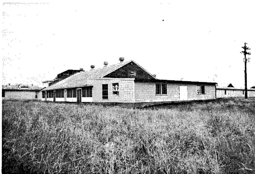
Figure 24. Building 809: Primer Loading Building.
