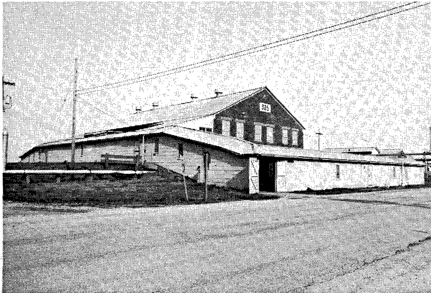
Figure 92. Building 325: Change House typical of Change Houses on every production line at Kansas Army Ammunition Plant with the exception of the 1200 line.
