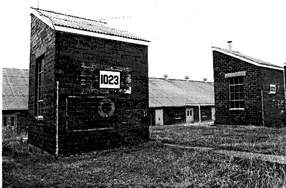
Figure 46. Building 1023 and Building 1022: Vacuum Pump Houses.
