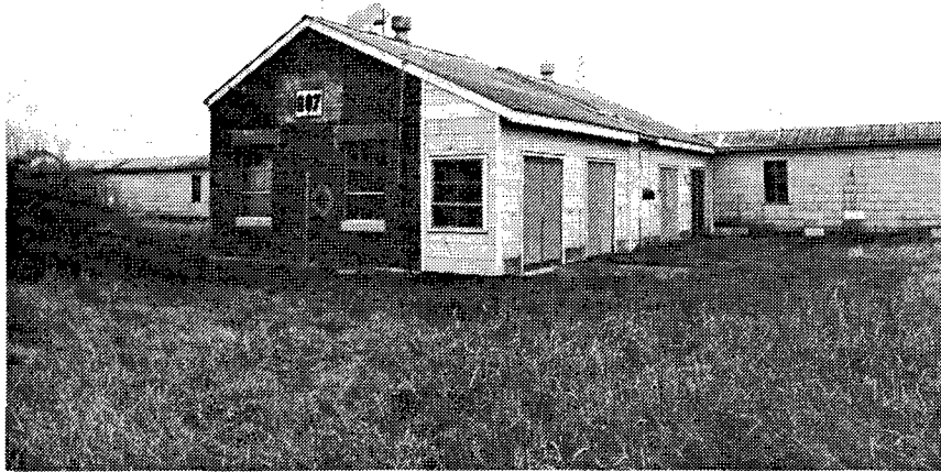
Figure 23. Building 807: Fan House.
