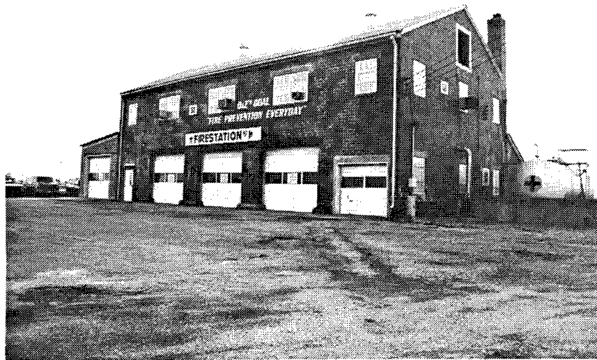
Figure 95. Building 52: Fire House.
