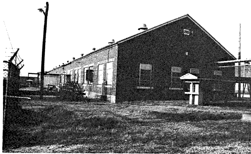
Figure 63. Building 203: General Purpose Administration/Maintenance Shop.
