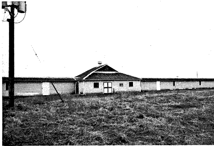
Figure 43. Building 1020: T.N.T. Screen House.
