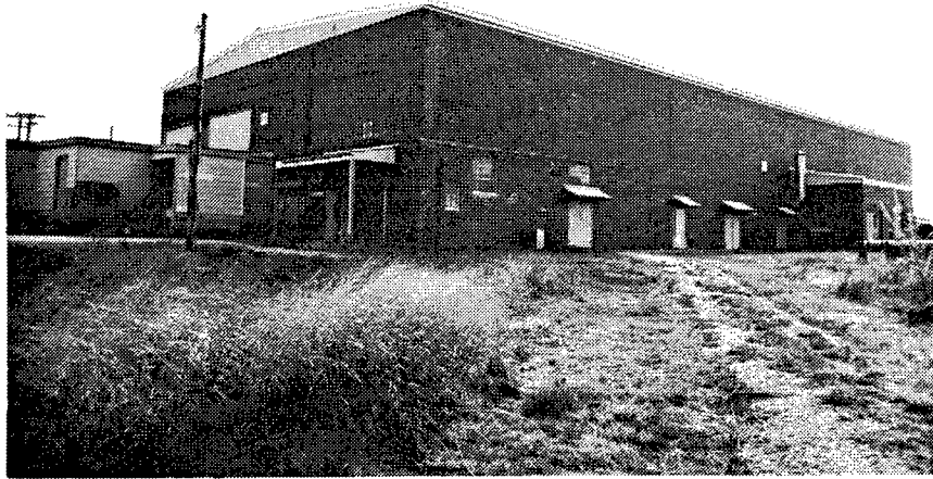
Figure 85. Building 1206: Neutral Liquor Storage.
