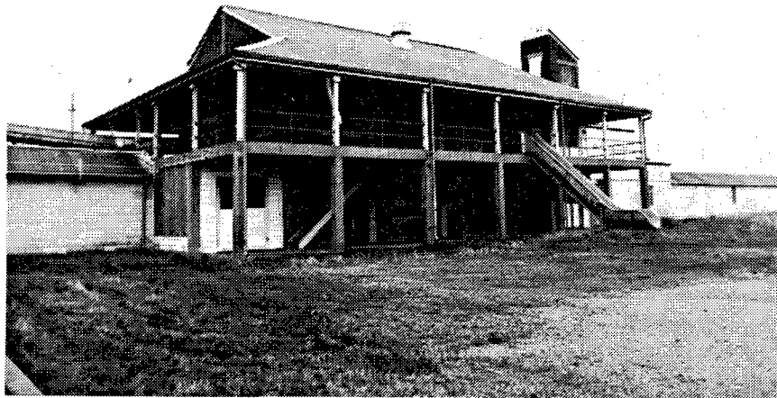
Figure 41. Building 1017: Screening Building.
