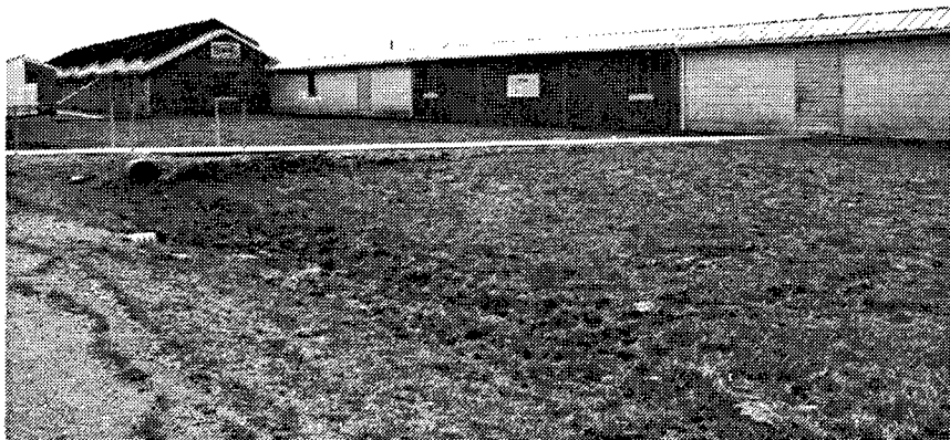
Figure 68. Between Building 504 and Building 507: This photo depicts a fire break in a covered walkway/transport way.
