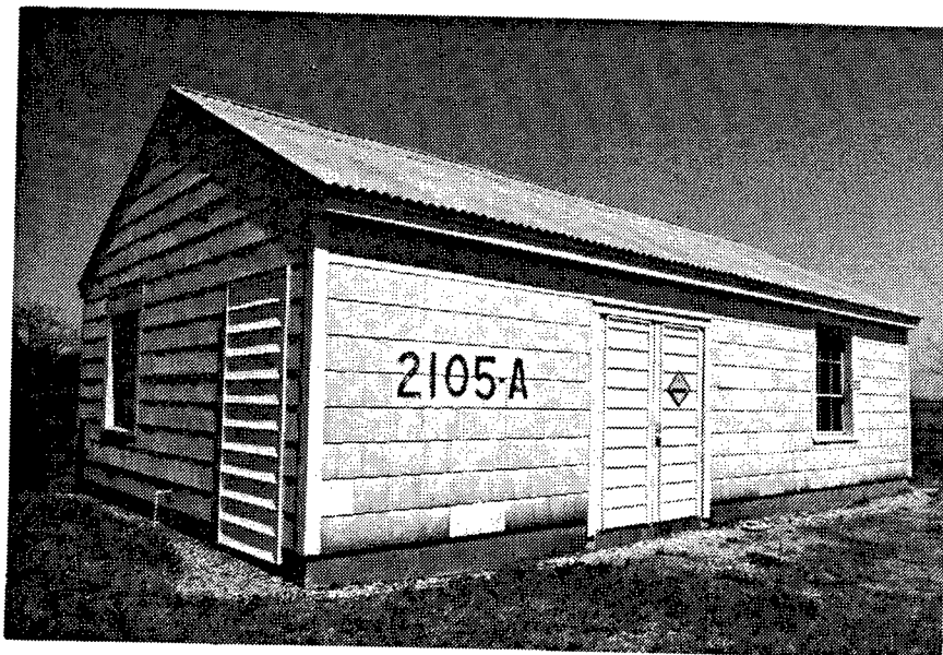
Figure 100. Building 2105A: Stone Quarry Pump House where water is pumped to and distributed by this centralized facility.
