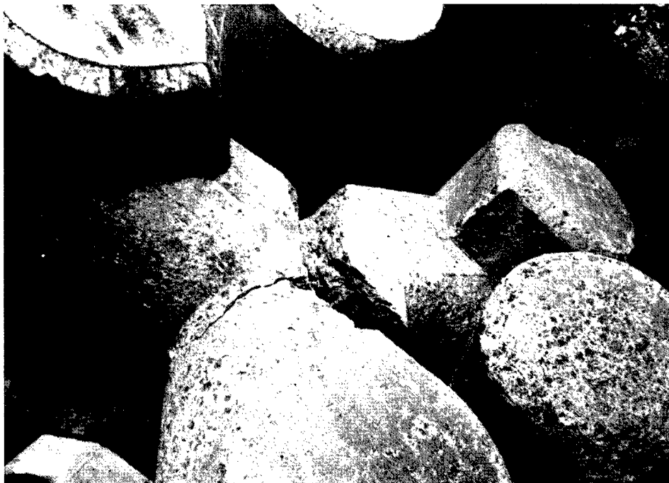
Figure 18. Tribar with break through center section of unit
