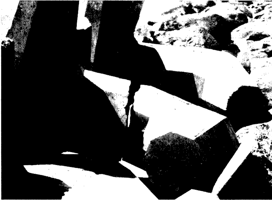
Figure 15. Dolos with mid-shank break
