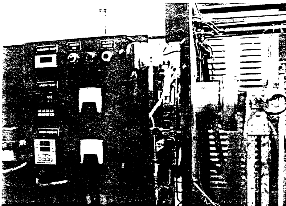
Figure 1. New gas heating system.
