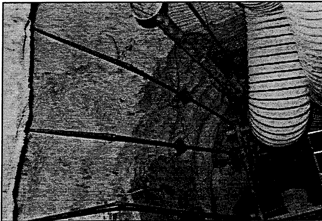
Figure D-24 Plug During Construction. Shown are Pressure Grout Pipes with Gas Checks ( Plates ) and 4" Dia. Bleed Lines
