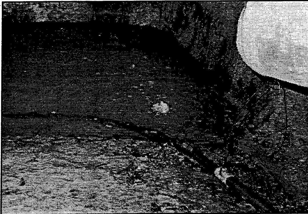
Figure D-28 Gas (Methane) Seepage at Sta. 18+50
