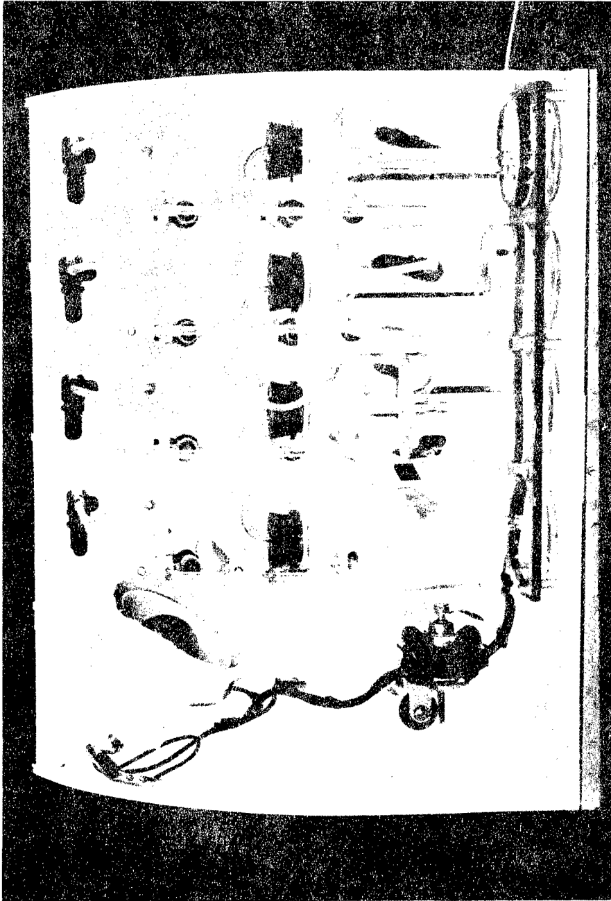
Picture No. 4 — Figure 3. Iron panel board (back view).
