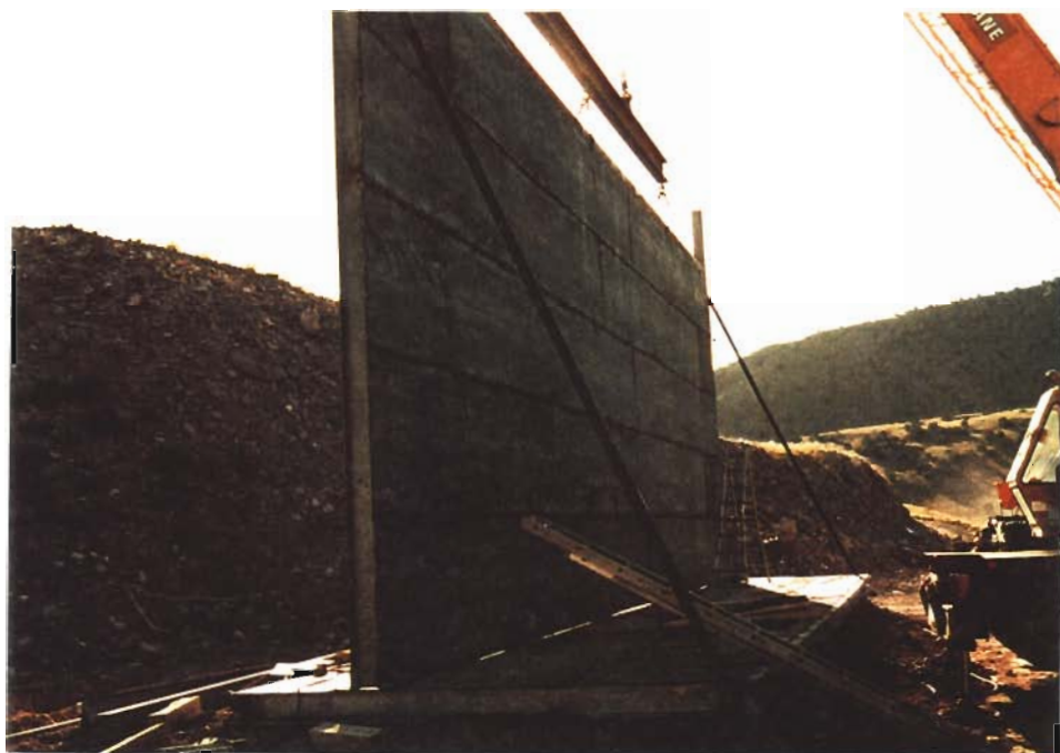
Figure 3: Witness Panel and Floor Plate. Oblique View
