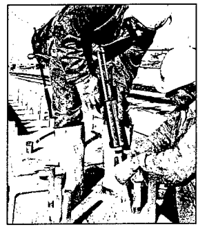
Anchoring highway sign trusses with Granite 5.
