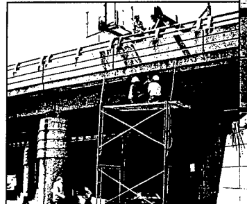
Bridge conduit and scaffold supports.
