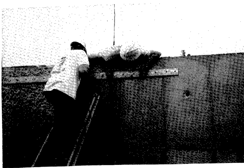
Figure 12. Profile pieces are used as a template to ensure correct positioning as anchor bolt holes are drilled in concrete
