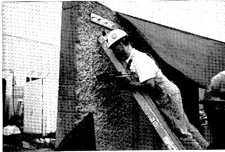
Figure 13. Injection of two-part epoxy resin for chemical anchor bolts
