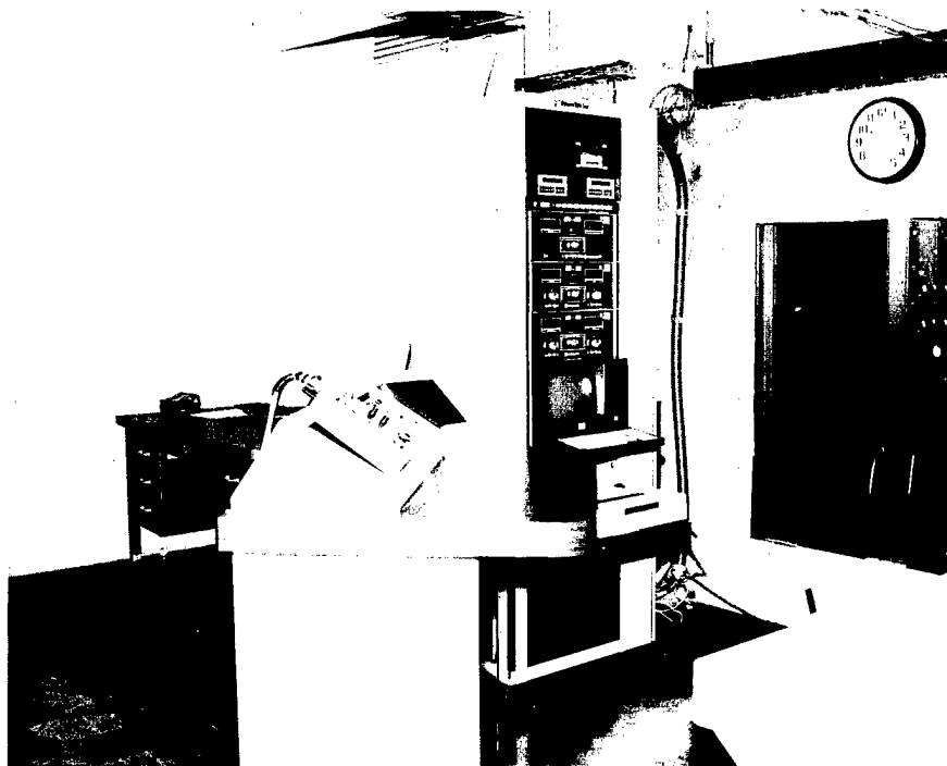
Figure 8 : Test Cell 5 Control Room and Instrumentation
