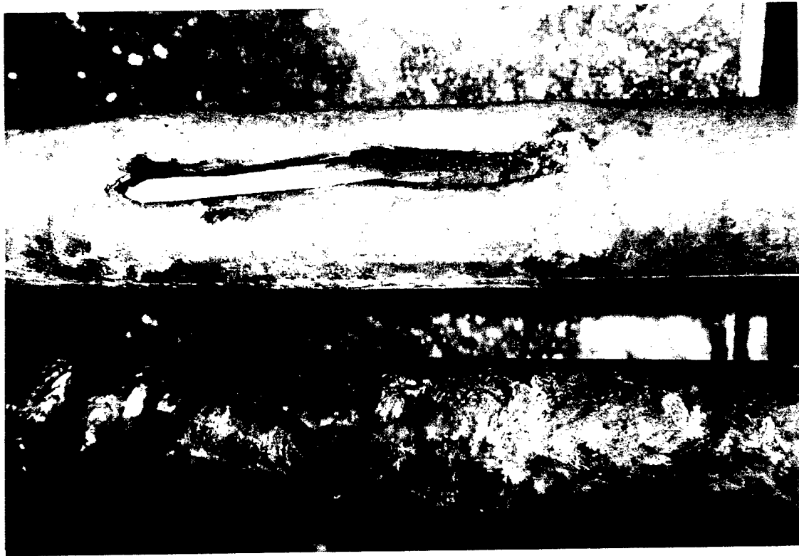
Fig. 5 - Chill water pipe rupture
